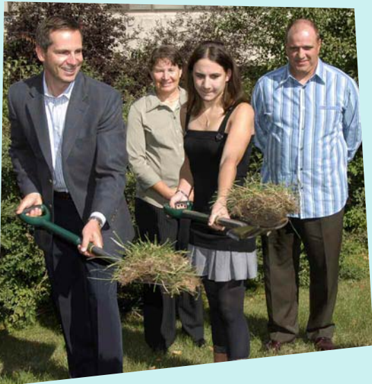
Premier Dalton McGuinty and Sarah Pion, former critical care patient, participating in the ceremonial ground breaking event to launch the construction of CHEO's new wing.
